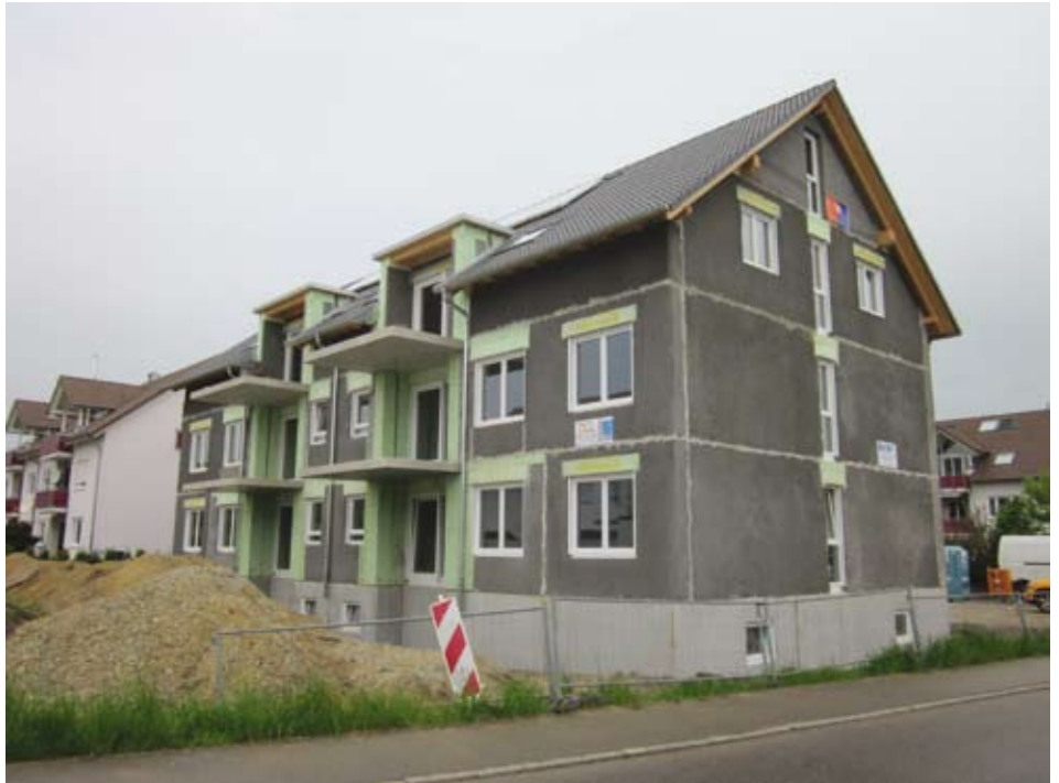
Construction of the new prefabricated house (Photo: Spedition Steinhart)
